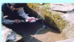
ひび割れ補修
